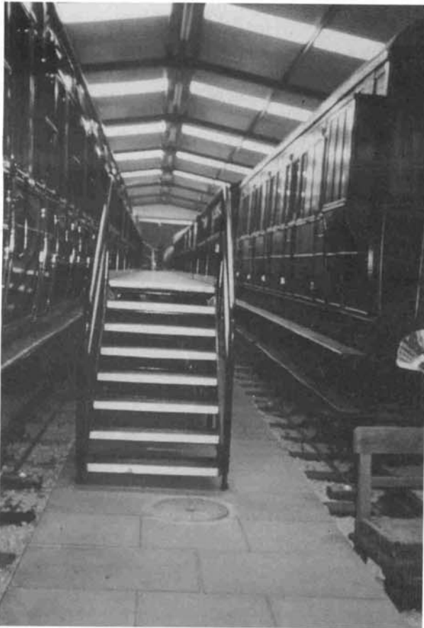
The project also includes replacing the present somewhat inadequate central walkway (seen above) with a purpose-built fully-accessible platform, allowing access to all carriages in the present building. As well as providing improved access for all, this will greatly improve safety – not the least by allowing us to dispense with the miscellaneous selection of access steps currently in use elsewhere in the Museum.
